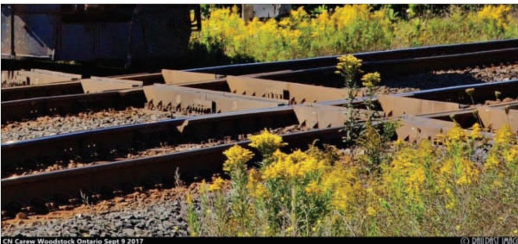
We've all seen railroad diamonds. In the photo to the left is a newer diamond where the single track is elevated above the double track mainline. Trains on the mainline can run at normal track speed since there's no break in the rails. The single track has a slow speed restriction. This type of diamond didn't exist in the steam era. On a recent MILW 261 4-8-4 excursion, the sand pipes got caught on the rail.
